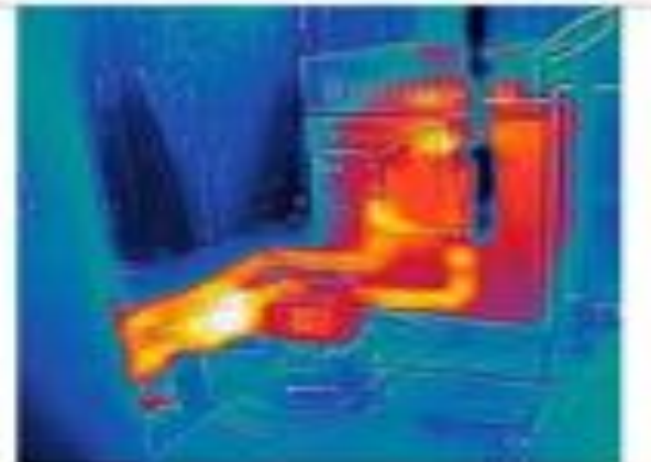
CHP system thermal image, heat loss from boiler which is off
